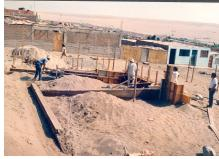
Figure 3: Group 8 Schoolhouse, Excavation and Formwork for the Perimeter Footing and Foundation. May 1988 (Photo: Pontificia Universidad Católica del Perú)
